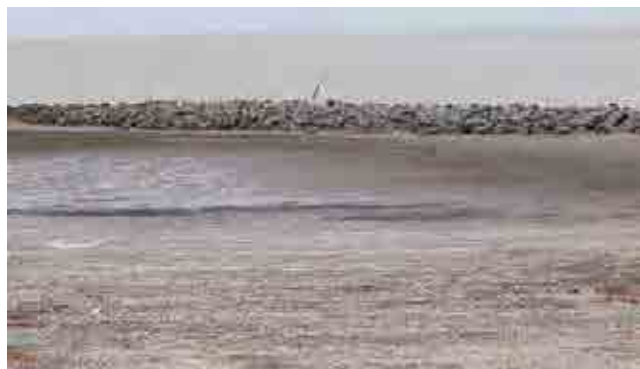
Figure 9 Rock dyke installed at the foreshore for erosion control
