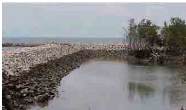
Figure 12 Rock dyke and groin constructed for erosion control
