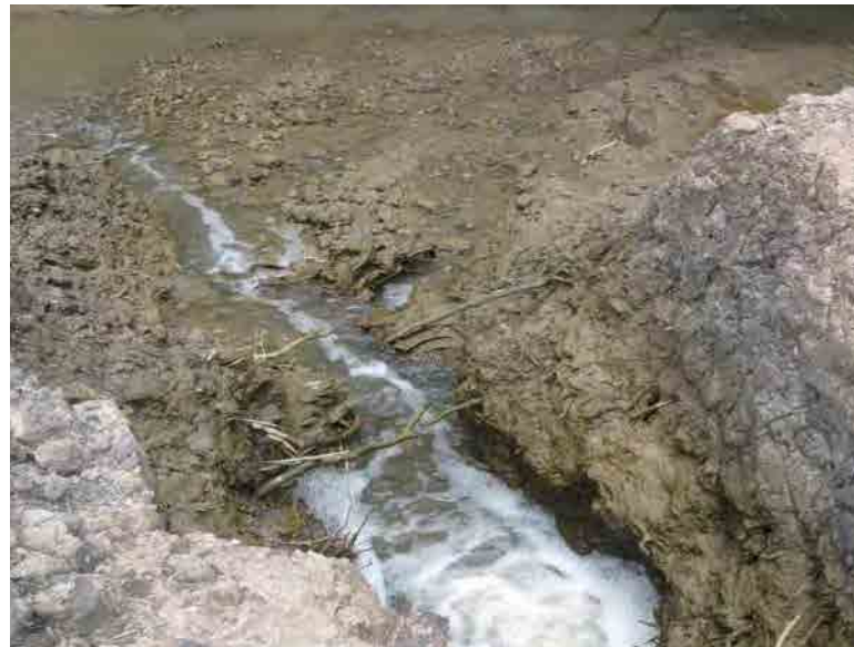
The bunds were breached at several locations to facilitate tidal flow.
