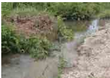
The bunds were breached at several locations to facilitate tidal flow.
