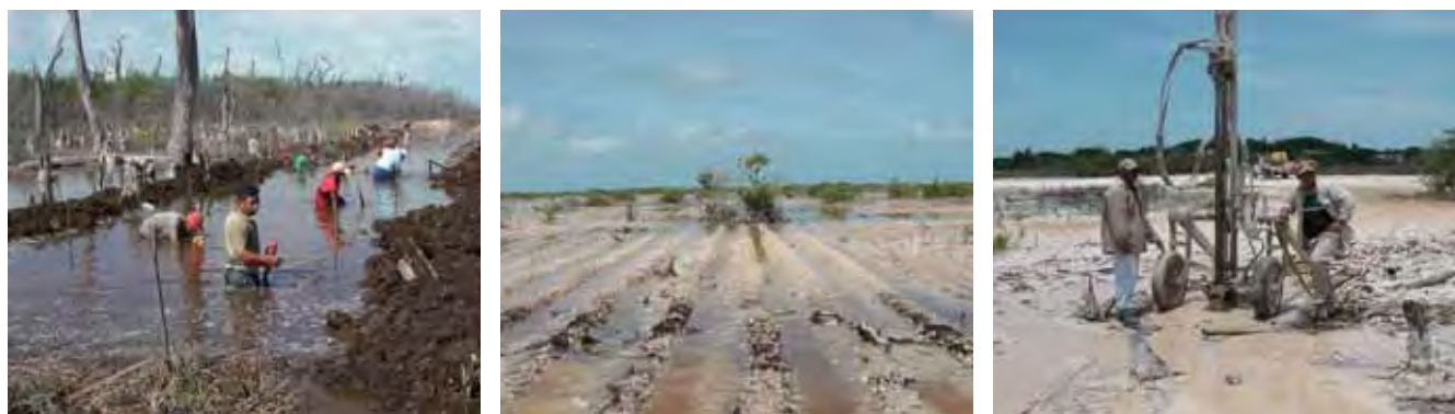
Figure 2.4 Digging a canal (left), trench and mound system (middle), and digging a well (right)
