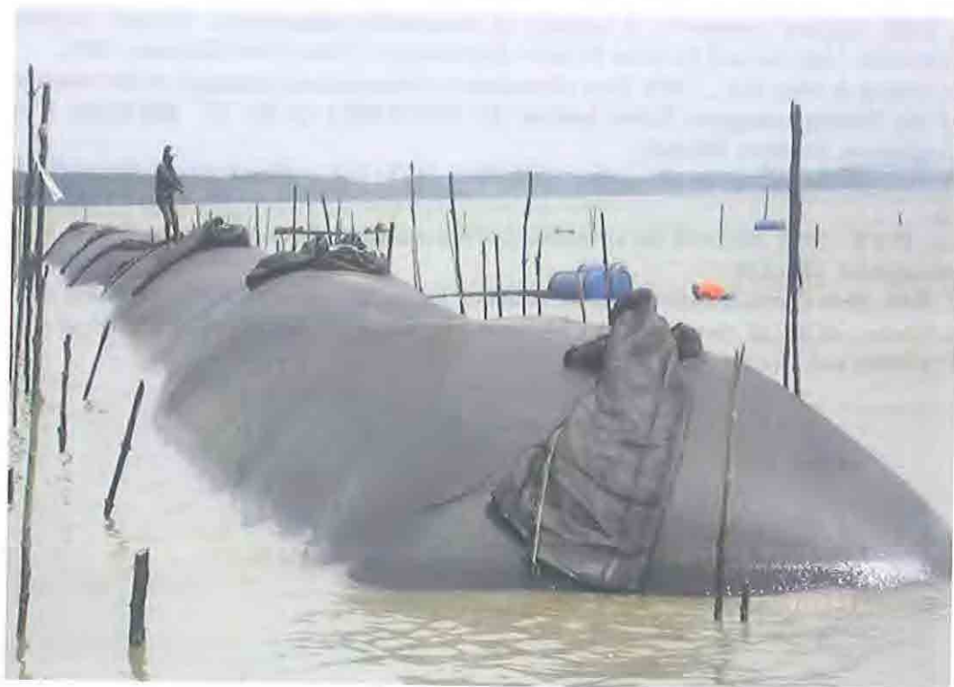
Fig. 1. A geotube being filled with sand during high tide
