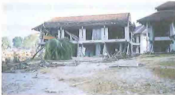
Structure type A: Damage level 2
