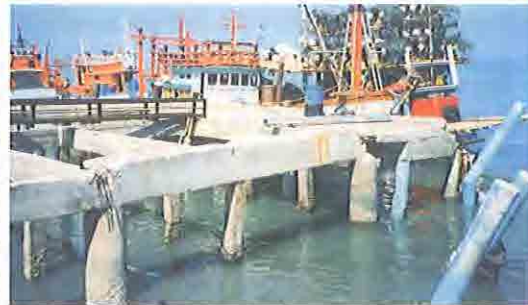
Structure type P: Damage level 2
